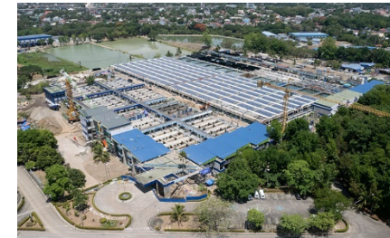
La Mesa Water Treatment Plant 1 Maynilad
