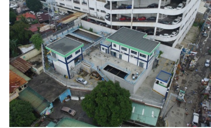
Tarayan Wastewater Treatment Plant World Bank
