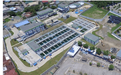
Parañaque Wastewater Treatment Plant JICA Sector loan
